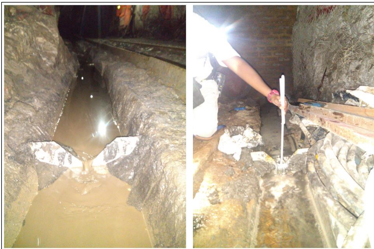
Figure 39: Photographs showing V-notch placement (left) and measuring (right) at 3/62E. The ventilation control wall made of bricks can be seen in the background on the right.
