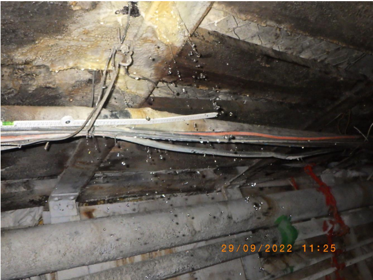
Figure 43: Photograph showing water flowing through steel sets supporting the Show-Stopper Fault. Note the white calcite precipitate covering the pipes and on the steel support.
